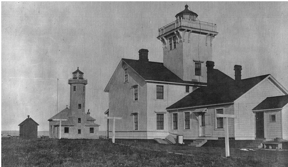
The original Point Wilson Lighthouse (foreground) with the new lighthouse in the background, 1914. USLHS archive photo.
