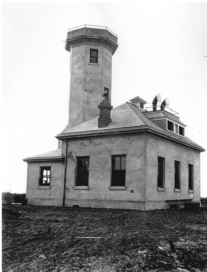
The new lighthouse under construction in 1913. USLHS archive photo.
